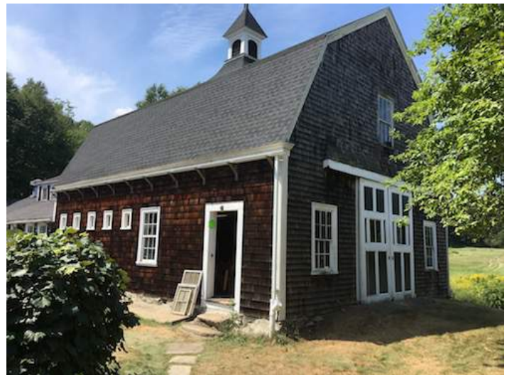
The gambrel-roofed barn. Photo by Christopher Martin, August 14, 2020.
